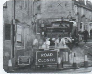
5 Repairs to streets and motorways. (4, 5)
